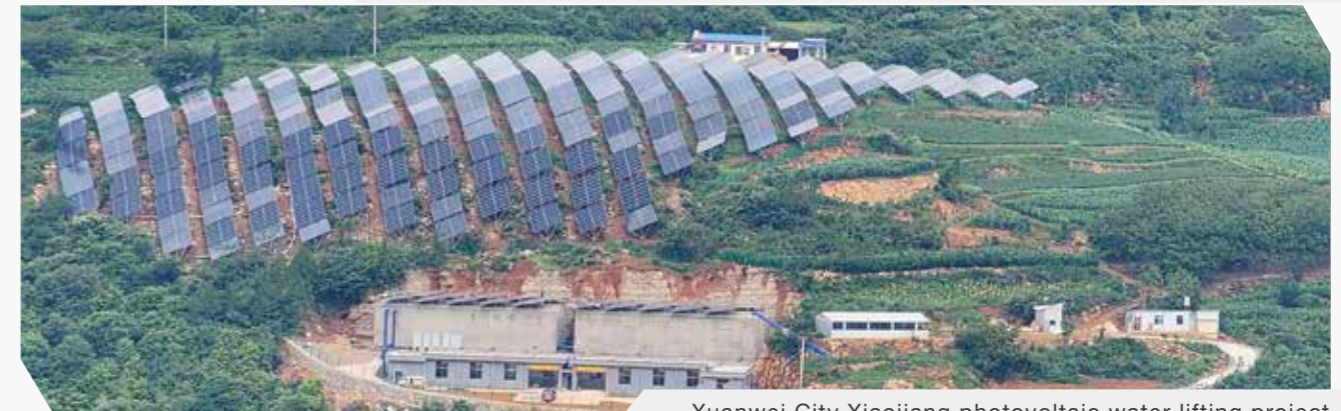
Xuanwei City Xiaojiang photovoltaic water lifting project
