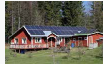
Areas without electricity or with insufficient electricity
