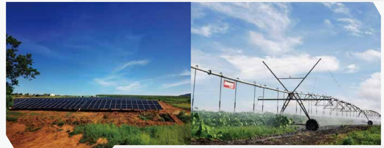
Africa · Zimbabwe 1.144MWp Wanjin photovoltaic power generation water lifting irrigation project
