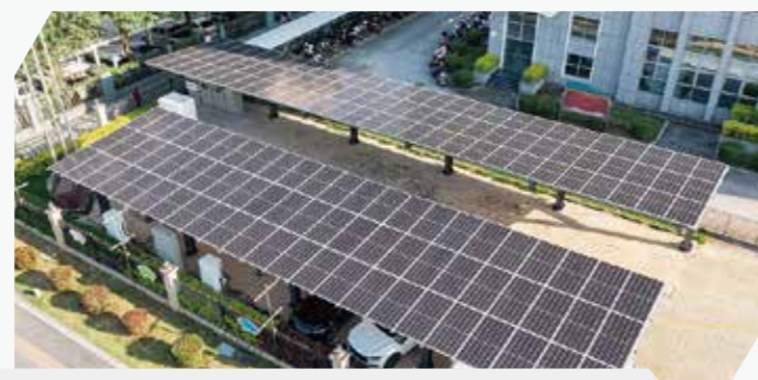
Zero Carbon Living Park Demonstration Project
