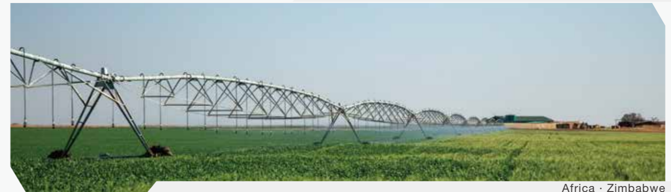
Africa · Zimbabwe 168kWp full photovoltaic direct drive high-power intelligent sprinkler irrigation system
