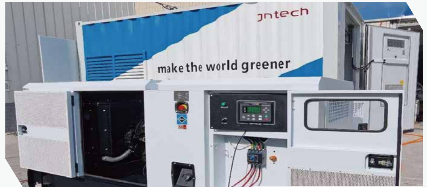
Congo Chaiguang storage microgrid system
