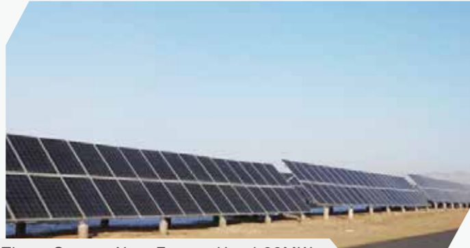
Three Gorges New Energy Hami 20MW power station project
