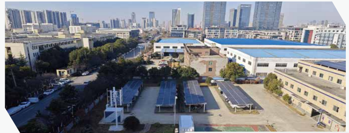
Hefei light storage charging power station project
