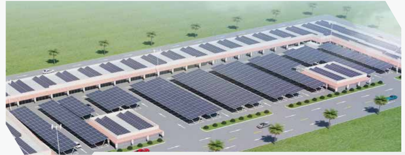
Las Vegas Scenery Storage and Charging Power Station Project (under construction)
