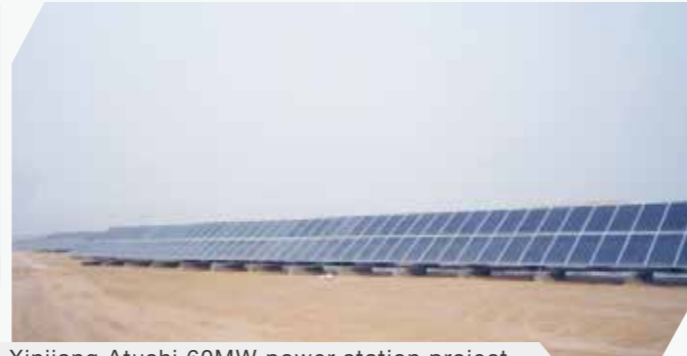
Xinjiang Atushi 60MW power station project
