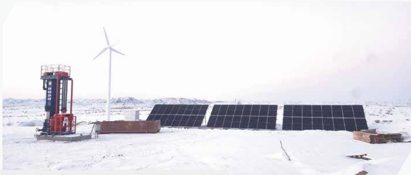
Xinjiang oilfield oil extractor micro-grid demonstration project
