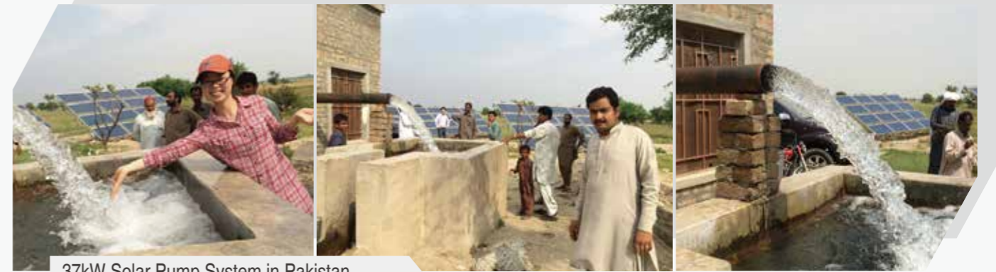
37kW Solar Pump System in Pakistan
